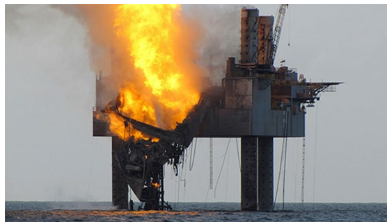
Hercules 265 Rig fire that caused a collapse of the drill floor and derrick after an explosion in the Gulf of Mexico, July 2013.
